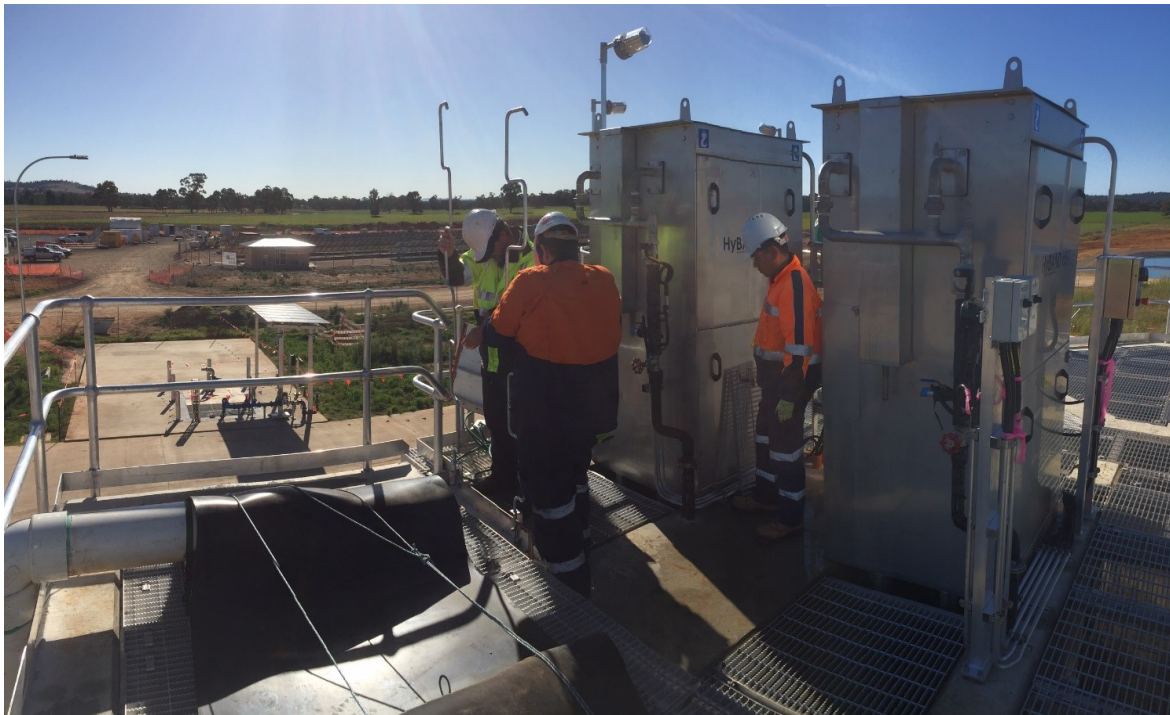
Figure 1. Commissioning of the upgraded STP (photo provided by Annalisa Contos)
